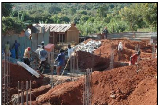
The foundation is dug and footings for the new building are put into place.
