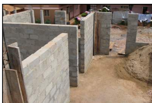
The walls for the new school building rise!
